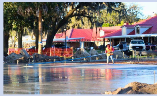
In Full Swing: Concrete Poured and Finished
