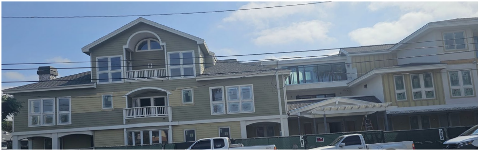
Orange County Ronald McDonald House under construction – Estimated completion July 2024
